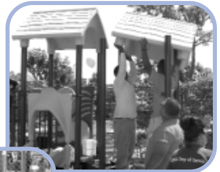
Above: Home depot volunteers putting the roof on the play equipment.
